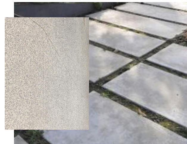
EXPOSED AGGREGATE CONCRETE PATIOS AND PAVERS WITH PEBBLE OR DECORATIVE PLANT INFIL
