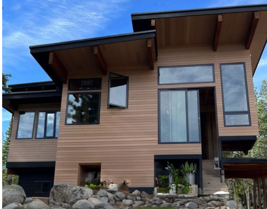
CEDAR SMOOTH FACE NATURAL TONE HORIZONTAL AND VERTICAL SHIPLAP WOOD SIDING 8 1/4" REVEAL, 1/4" GAP
